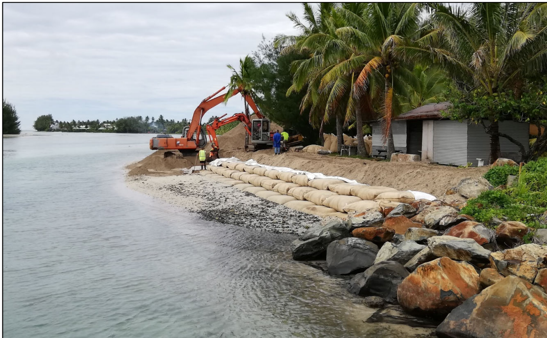
Figure 1: Construction of Geobags at Avana in November 2011, photo 23/11/2020.
