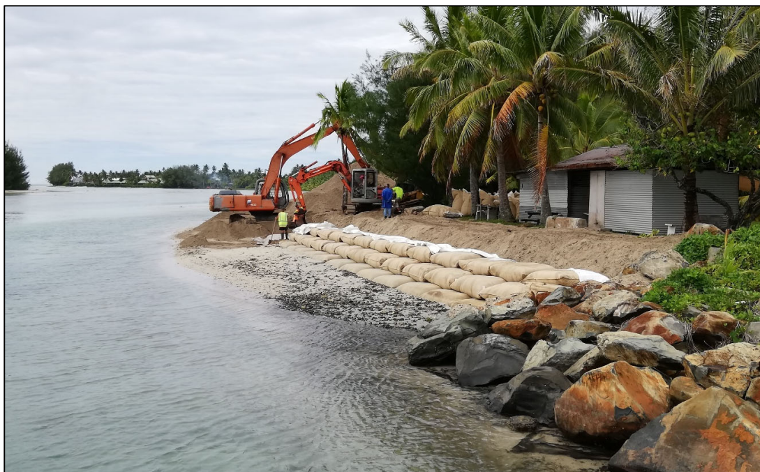
Figure 2: Construction of Geobags at Avana in November 2011, photo 23/11/2020.
