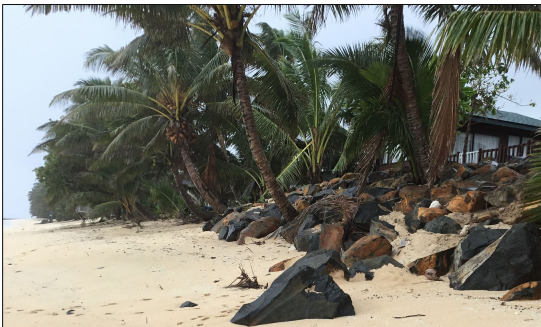
Figure 1: Recent rockwall construction at the adjoining property of Tuingariki Short, photo 08/05/2023.
