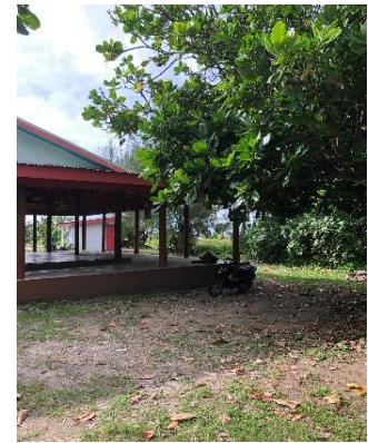
Figure 16: Overgrowth of trees is a hazard waiting to happen, in this case over the Are
