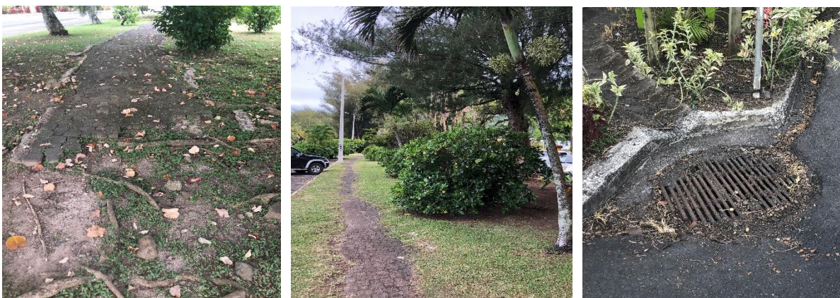
Figure 9: Some of the landscape characters identified; L-R. Damaged foot path by roots, footpath requiring maintenance and drainage systems around gardens.
