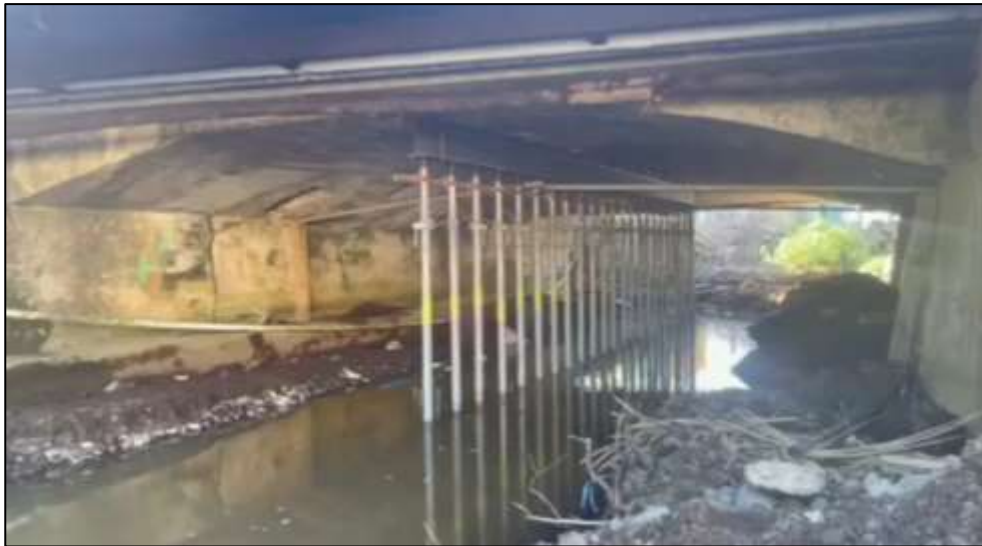
Figure 2 Temporary steel bracing under the Empire Bridge (August 2021)
